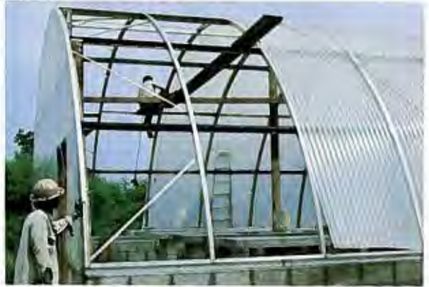
Greenhouse construction in progress
