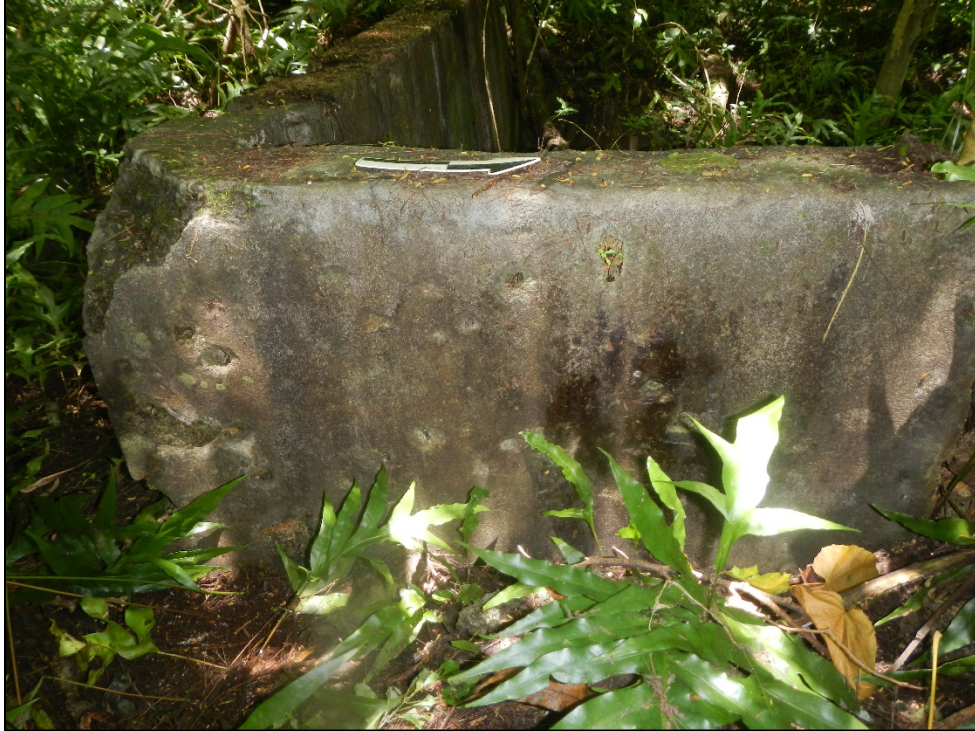
Figure 5: Okinawan cistern with bullet holes and concussion spalls. Site CHT-11. (Source: Dixon et al. 2019.)
