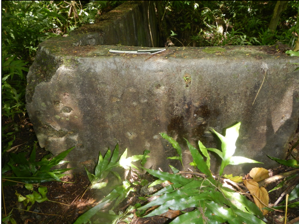
Figure 5: Okinawan cistern with bullet holes and concussion spalls. Site CHT-11. (Source: Dixon et al. 2019.)
