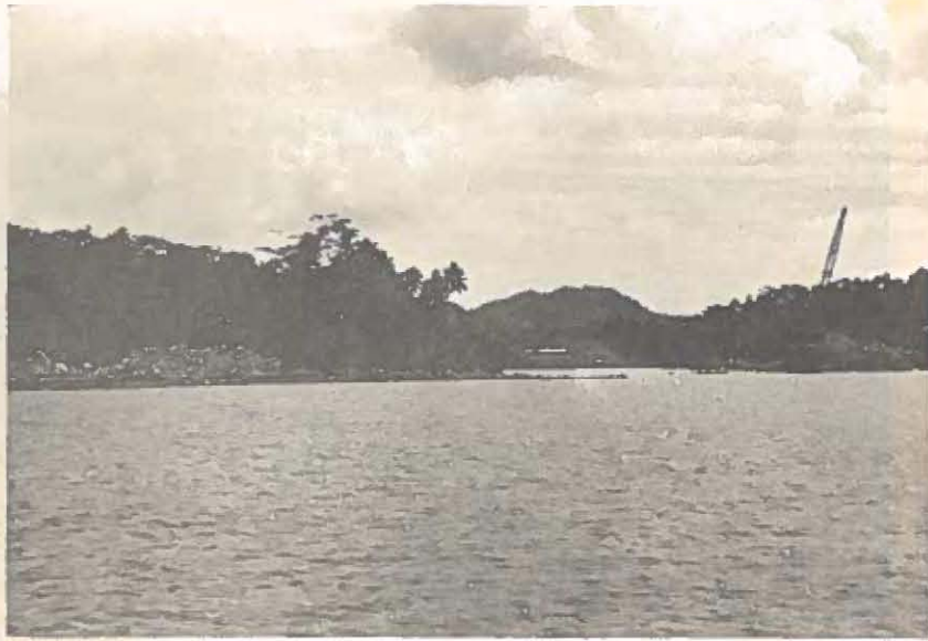
Fig. 1. Site of dredging operation at south end of Tuanmokot Channel.
