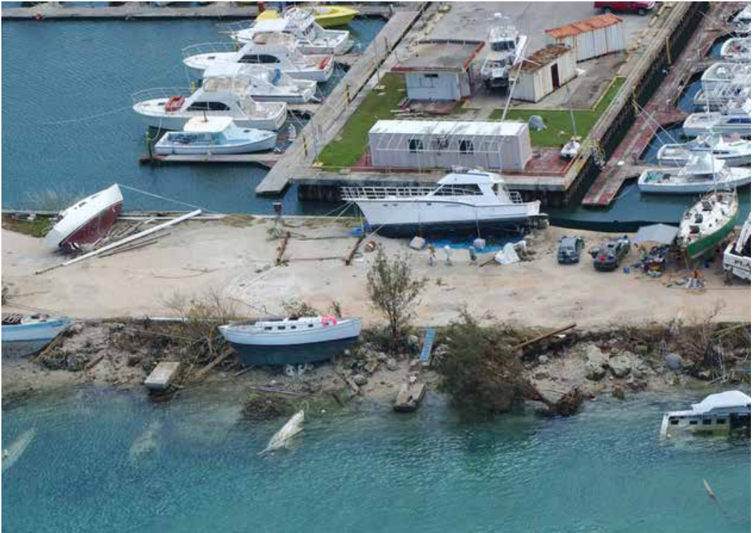
Figure 3.2. Boats damaged and submerged after Supertyphoon Pongsona passed the island in December of 2002.
