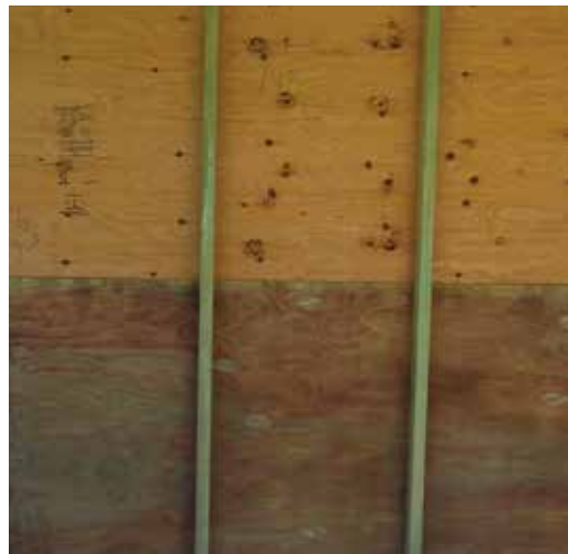
Figure 2.27. For larger windows, such as this sliding glass door, two 2x4s face outside and then are oriented with the narrow end against the plywood. The fastening screws attach from the plywood into the 2x4.
