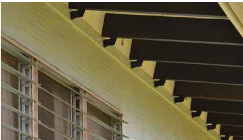
Figure 2.20. With the proper trim, the HPT clips can be installed as shown. Every rafter is connected to the wall in a visually pleasing way. Adding trim is not hard to do but will double the installation time. Two people working on this project could probably complete it in about three to four days.
