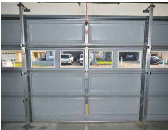
Figure 2.29. Vertical braces, like these, can be deployed during high wind events to strengthen the garage door. The braces are secured from the header over the garage door to the fastener installed in the concrete floor. Deployment and breakdown are about ten minutes each. The windows have been covered with a laminate film.
