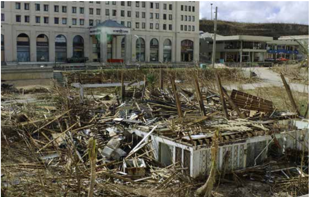
Figure 2.5. Extensive damage in Tumon caused by Super Typhoon Pongsona. Deciding to reinforce your home and prepare your property for a storm is a good idea. Storms can be intense and potentially deadly. Take the time to prepare your family and decide if you would look for shelter somewhere other than your home.
