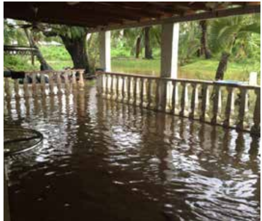
Figure 5.1. A porch on Guam is inundated with flood waters after heavy rains associated with Typhoon Halong in December 2014.
