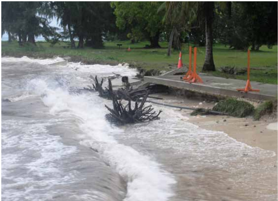
Figure 1.8. Storm surge eroding the shoreline at American Memorial Park, Saipan. Source: Robbie Green, Department of Coastal Resources Management, CNMI.
