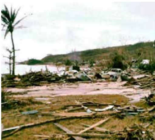
Figure 2.1. Wreckage from Pongsona in 2002. Source: FEMA.
